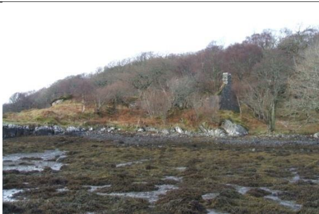
A two-floored cottage. View from South. 66630/74304.
